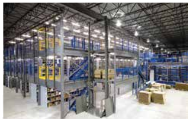
STORAGE PLATFORM WITH NO-BOLT SHELVING
