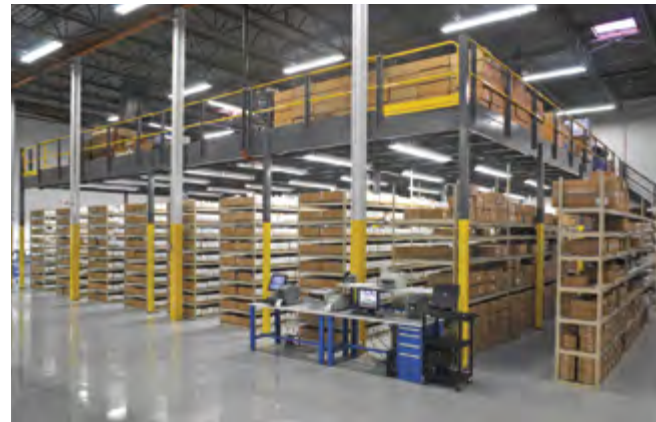
STORAGE PLATFORM WITH SHELVING
