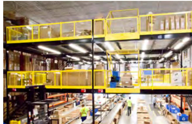
STORAGE PLATFORM WITH PACKING STATIONS
